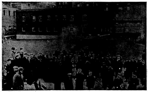
Packinghouse workers seized the plant during their recent strike and left only when Governor Olsen dispatched troops and threatened to drive them out.
